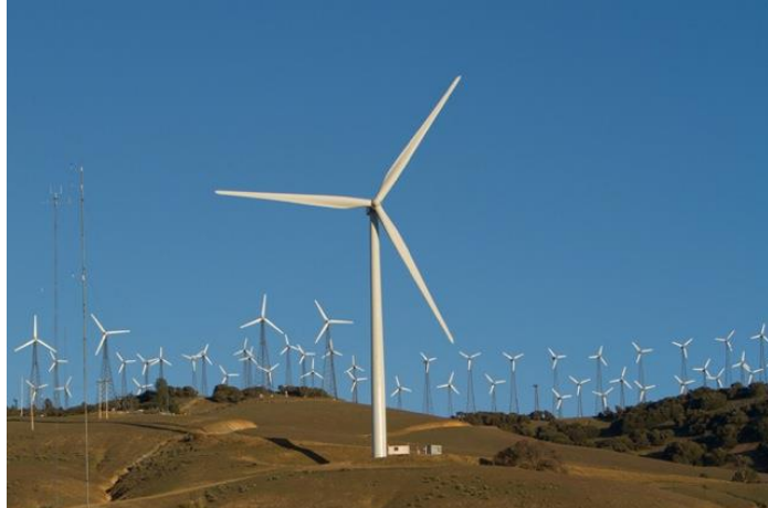
Typical US wind farm that can store electric energy using green energy lithium storage solutions.
