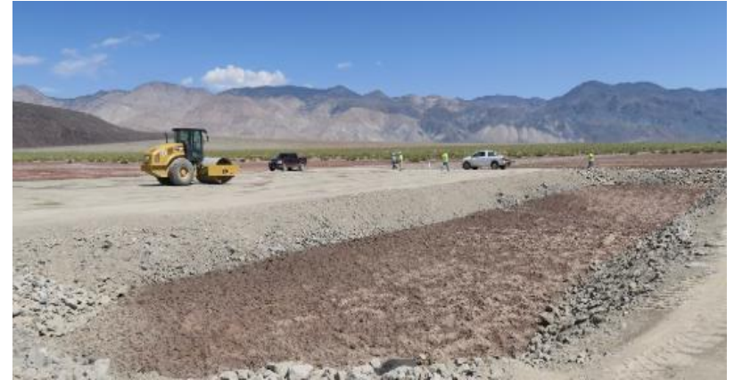
Drill Pad #1 and Associated Sump
