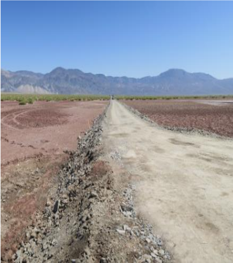
Access Road to Drill Pad #1
